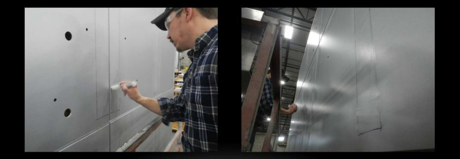
ACM plates shipped with factoryapplied TESA ACX adhesive Numbered ACM plates are test-fitted to each coordinating panel
